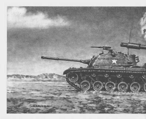
but it lacked sufficient firepower and protection. The M26 heavy tank increased firepower and armor at the expense of mobility. It suffered from being under-powered. Its replacement, the M46, featured a new engine, cross-drive transmission, a bore evacuator, and fire control and suspension improvements, modifications that resulted in better overall performance, but it was still not an ideal heavy tank.<sup>3</sup>
